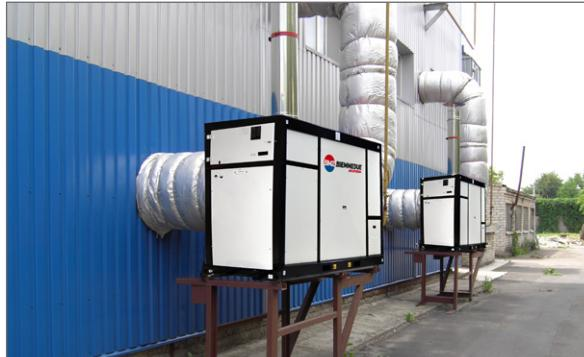
**SCUDO - BASE FRAMED INDIRECT COMBUSTION SPACE HEATERS WITH CENTRIFUGAL FAN**
